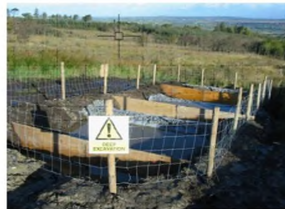
COMPLETED SETTLEMENT POND SYSTEM SCALE: NTS
